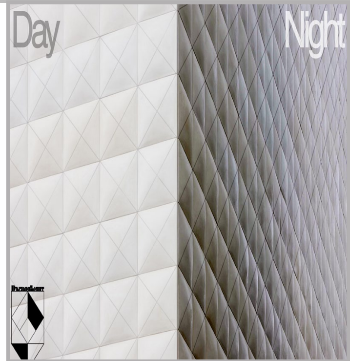
Fig.64. Day and night. The facade system has the ability to portray differnt things depending on its environment
